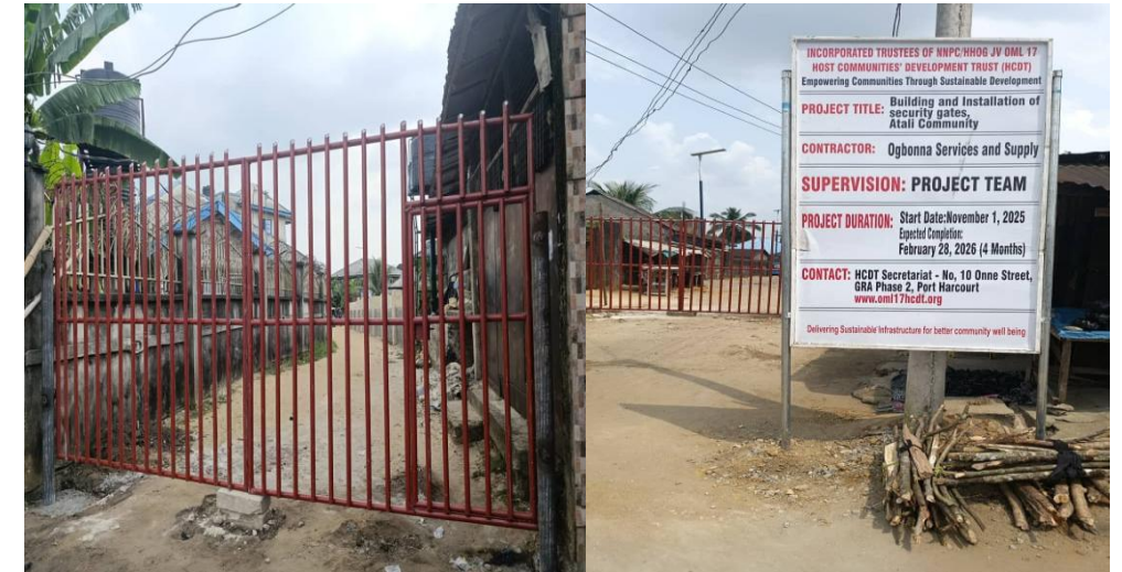
Installation of Security Street gates, Agwarire
