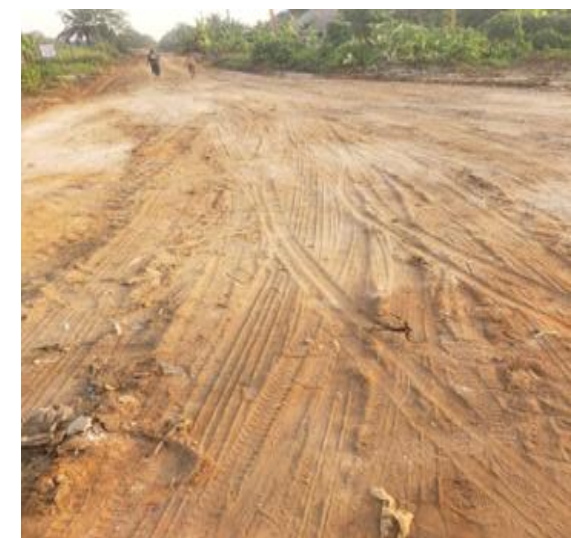
Road Grading, Isu
