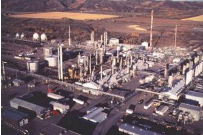
GAS PROCESSING PLANT
